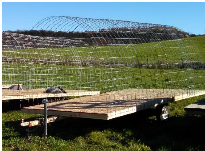
Single Deck portable shelter prior to plastic covering
